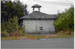
The old fire hall on Summit Street. Many years of neglect had reduced the building to the demolition stage. The wooden driveway ramp had rotted out to where it was unsafe to walk on. Some of the large wooden upright timbers had settled and the building had developed a pronounced list to the north.
